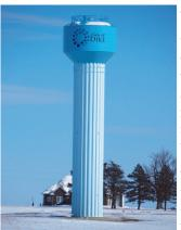
The City of Dike officially connected to CIWA on November 1, 2014, upon completion of a new 300,000 gallon water tower and 10" transmission main upgrades necessary to serve the city.
